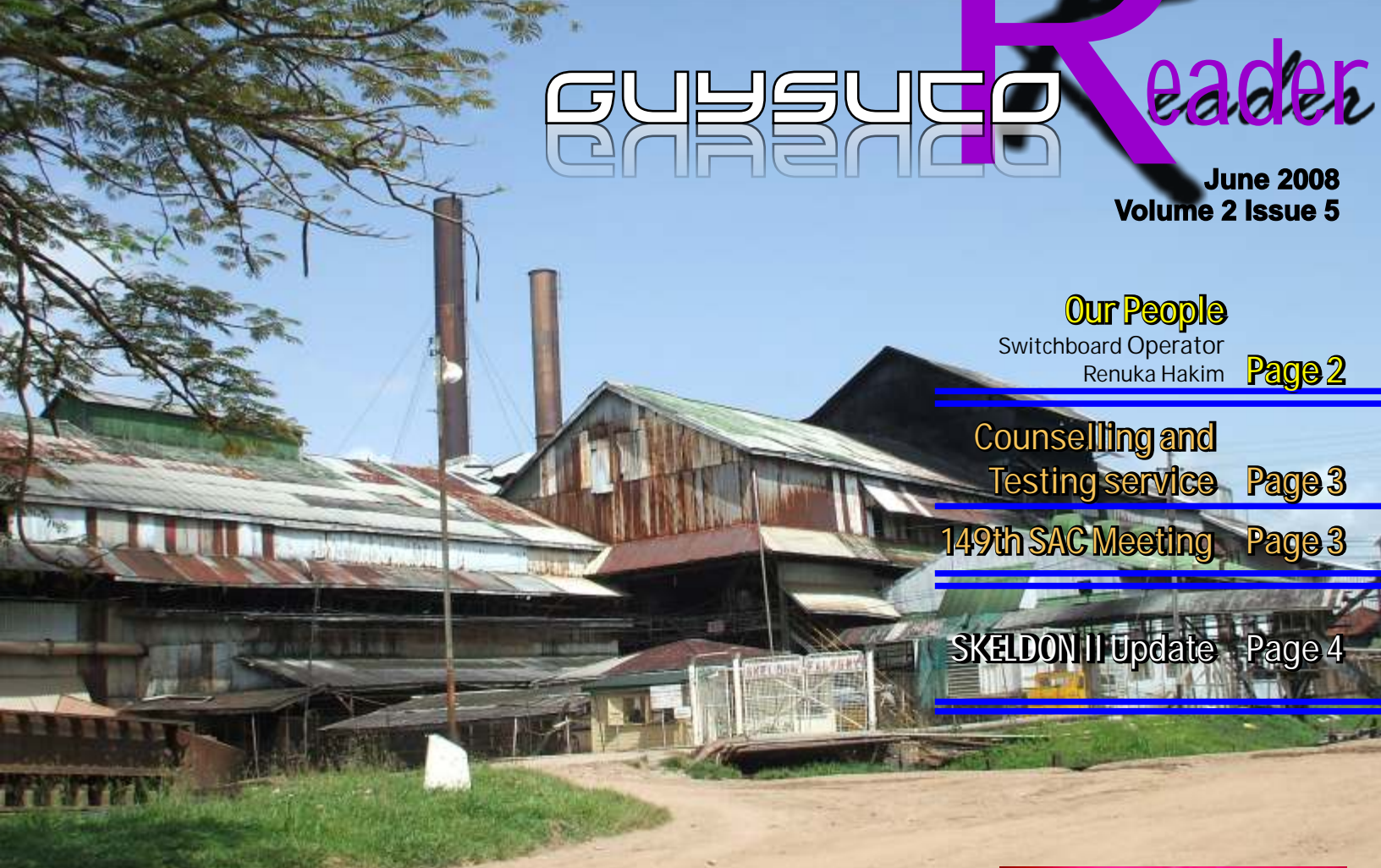
The former Skeldon Factory
